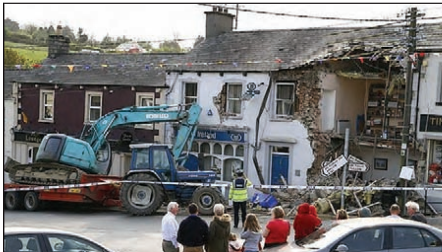
Now that really is a hole in the wall!: The aftermath of an attempted robbery of an ATM machine from the Bank of Ireland Branch in Tinahely, Co. Wicklow (Photo: Michael Kelly).
